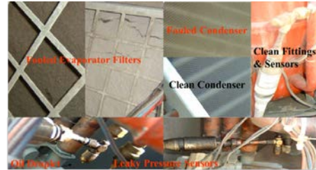
Figure 2. Common faults in a HVAC system
