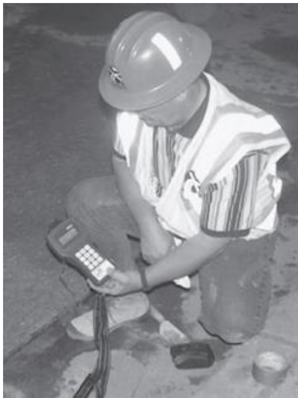
Figure 6: Concrete maturity monitor
