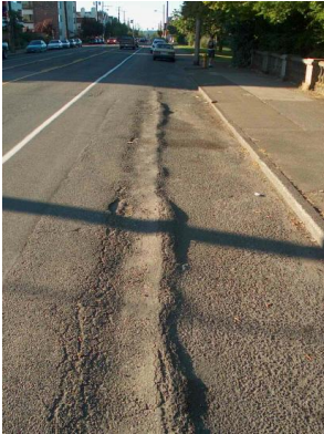
Figure 4: Rutting (Rutting, 2022)
