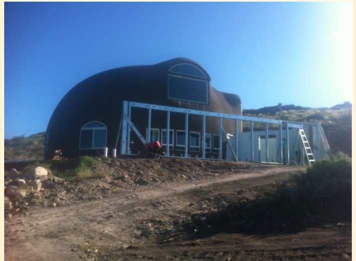
Dr. Lionel Hewett's house at Colorado, under construction
