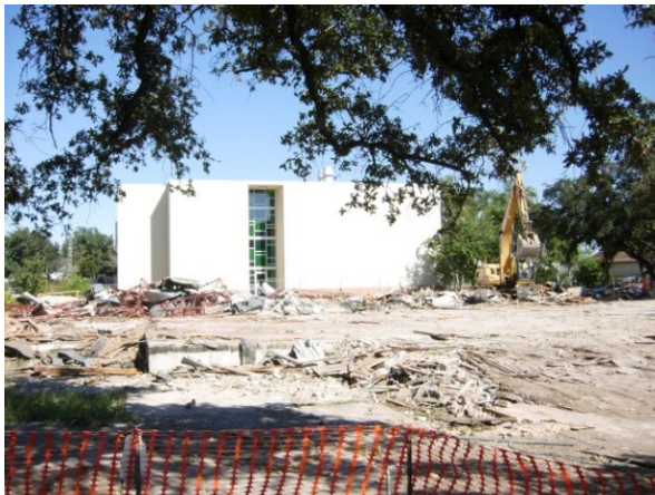
From behind the rubble, the new appears
