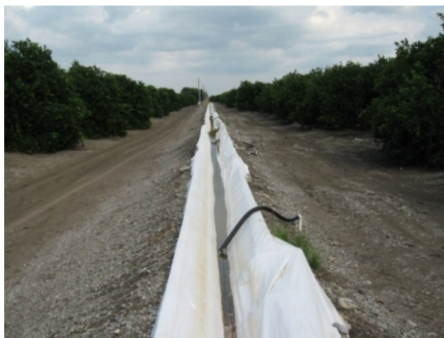
Figure 1 Plastic lined canal on Carlos Montemayor's 'Valencia' Orchard in Mexico.
