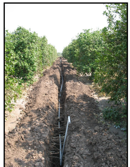
Irrigation Line being installed
