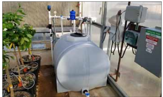
New fertigation system installed in Stephenville back up screenhouse
