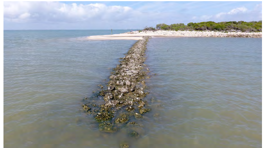
Example Artificial Reef Helps to Dissipate Damaging Energy from Storm Surges
